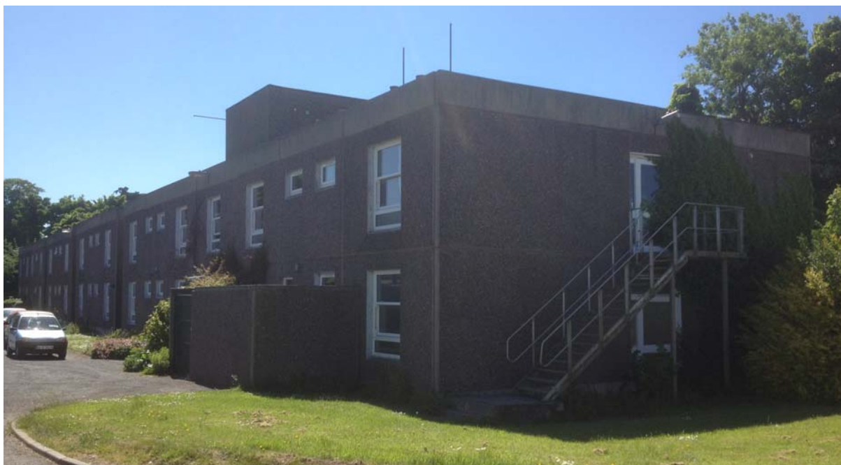
Figure 8: View of the Southeast facade [MosArt, 2013]
