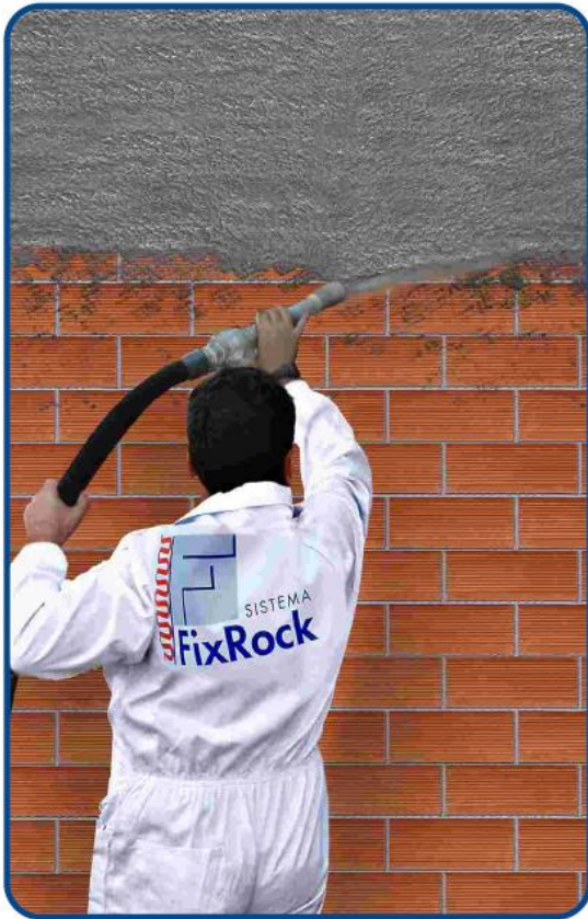
Figure 1: Rockwool installation from the inside
