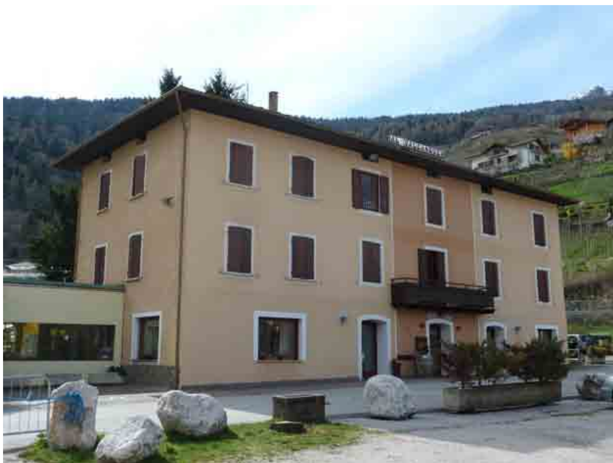
Figure 1: The existing building [ZEPHIR, 2013]
