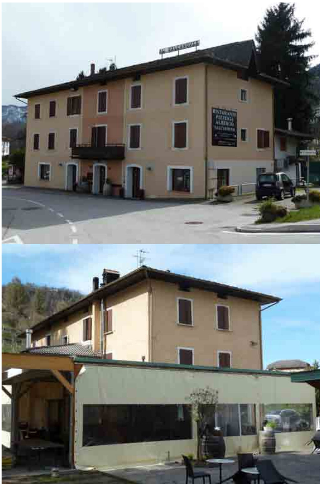
Figure 2: Pictures of the existing building. Top: north view. Bottom: south view. [ZEPHIR, 2013]
