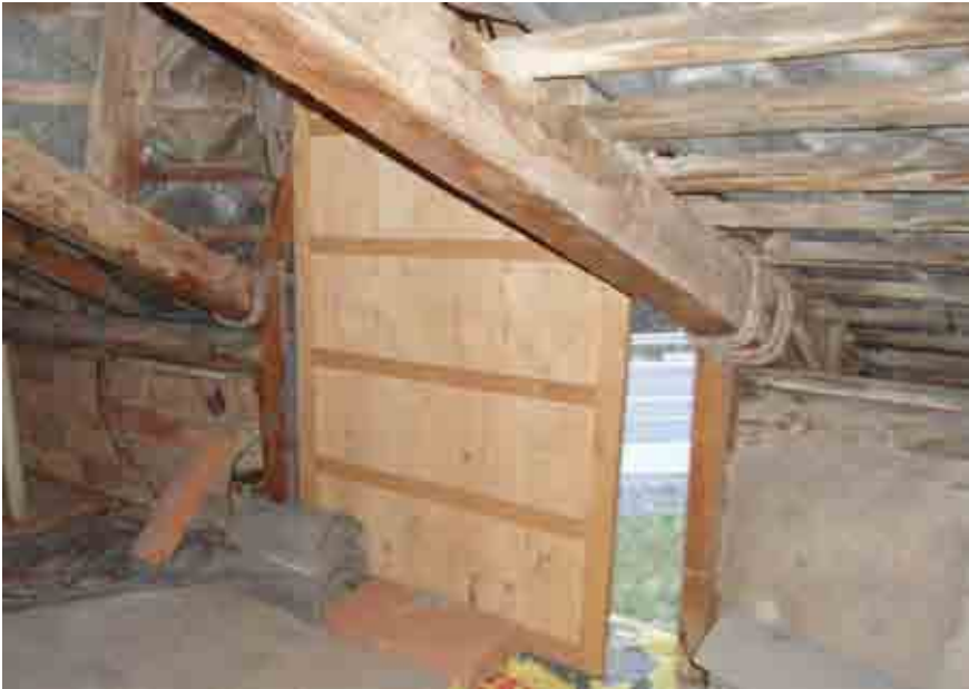
Figure 6: Roof of the existing building [ZEPHIR 2013].
