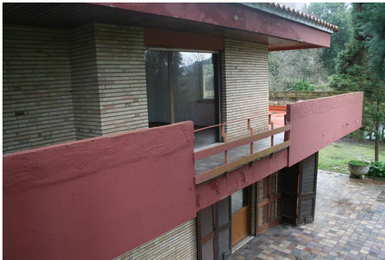
Figure 1: External views of the existing buildings [AIU ArquitectUra]
