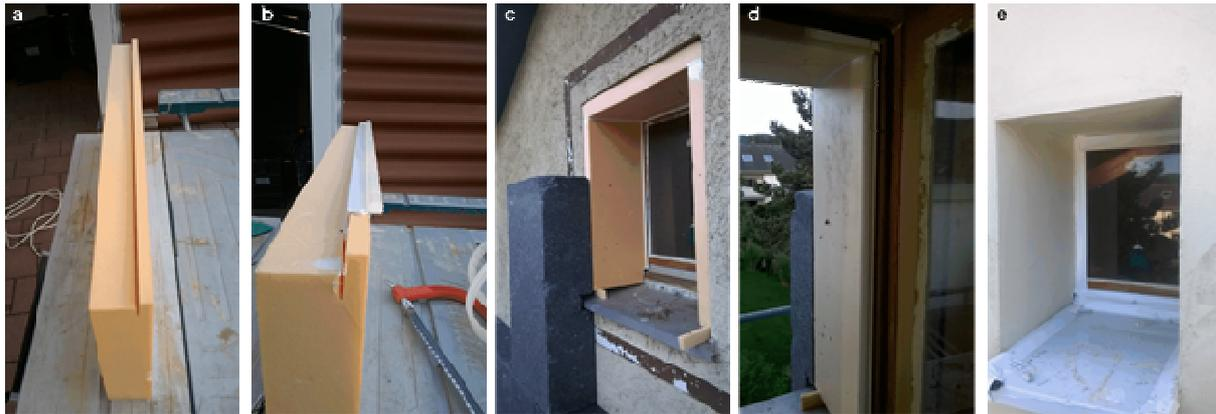
**Figure 3:** Insulating sash and reveal: a) XPS board notched to size; b) PVC profile inserted with hose gasket glued on; c) inserted in the reveal; d) interior view; e) exterior view after plastering
