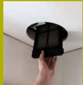
Filterwechsel | Filter replacement
