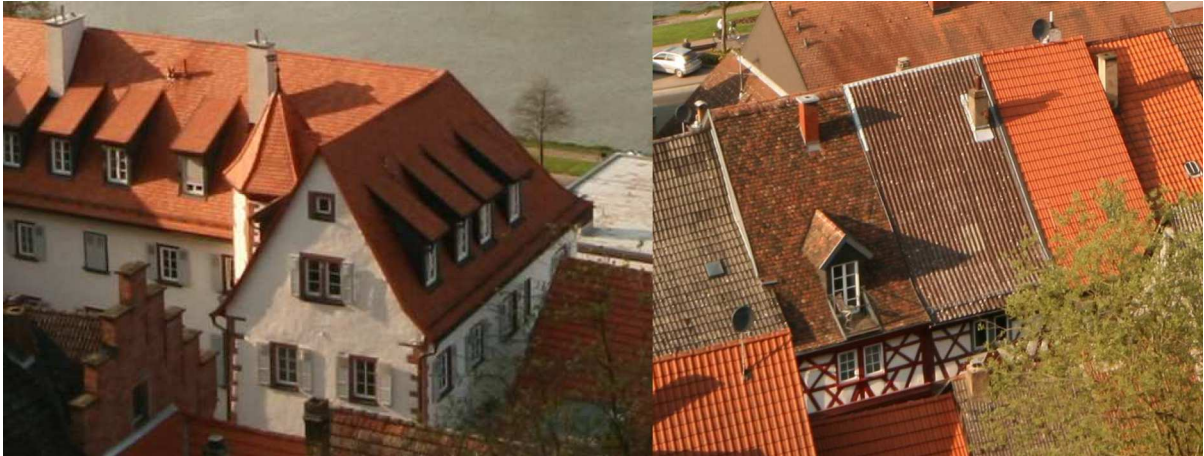
Figure 5: Typical Franconian buildings in lattice construction with and without render finish, Miltenberg, Germany. Source: Jose Alonso
