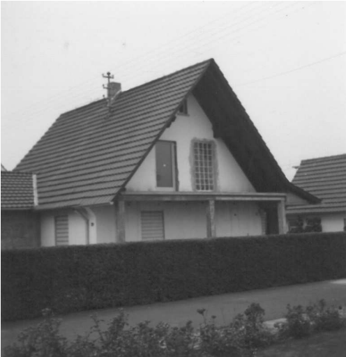
Figure 6: Additions to the original design. Balcony and glass block element. Source: Karl Theumer
