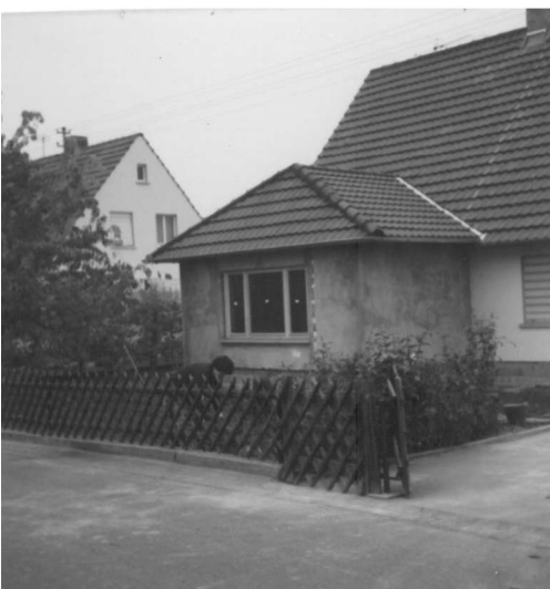
Figure 8: Additions to the original design. Living room extension. Source: Karl Theumer
