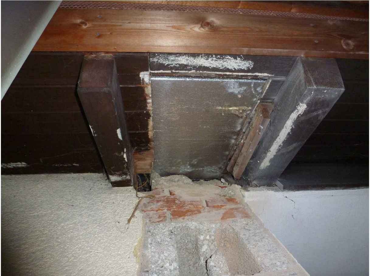
Figure 11: Eaves connection is not airtight. Provision should have been made to close the leakages. Instead, the timber (not airtight) joints were sealed. Source: Karl Theumer
