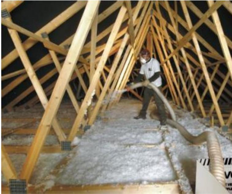
Figure 14 Blowing the Comblissimo glass wool
