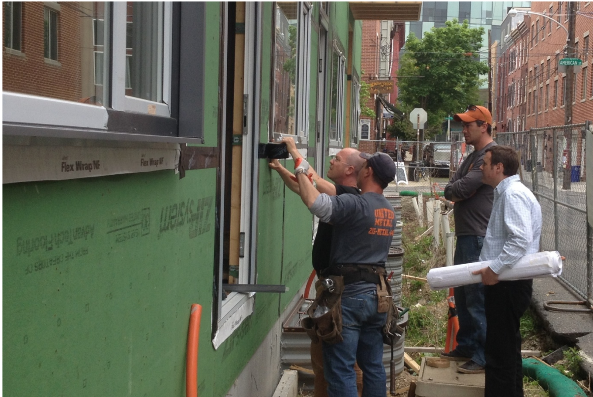
Figure 2: On site airtight taping demonstration
