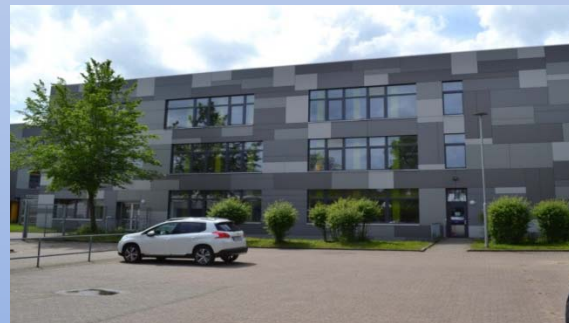
Renovation of a school campus in Aachen. Primary energy use reduced from 240 kWh/m 2 /year to 78 kWh /m 2 year
