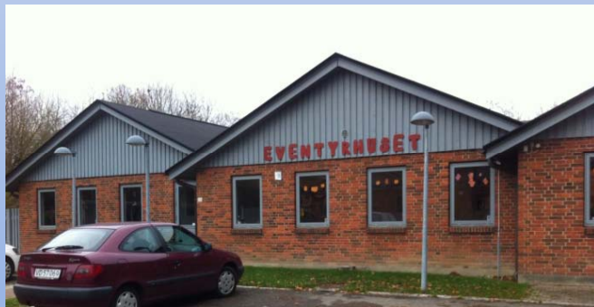
Renovation of a kindergarten in Denmark Primary energy used reduced from 224 kWh/m 2 /year to 103 kWh/m 2 /year
