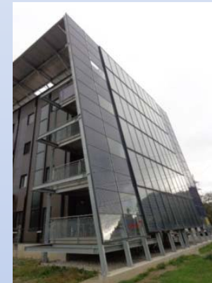
Renovation of a residential building in Kapfenberg (Austria) – renovated to 85% site energy use reduction
