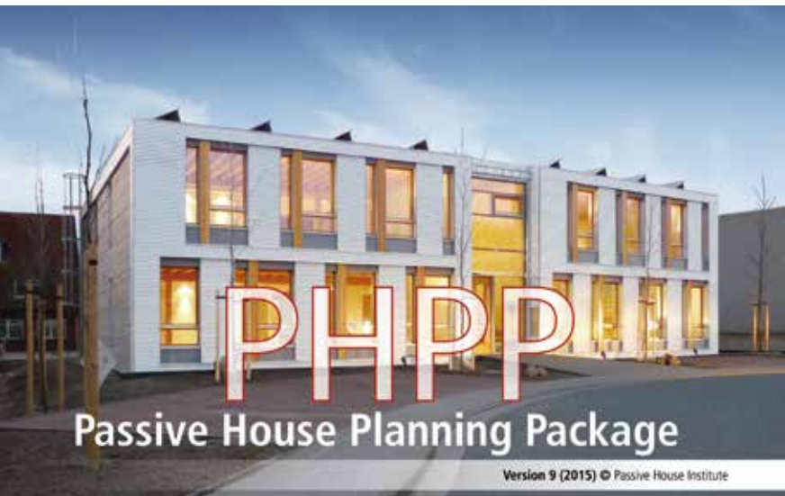
Figure 4: Version 9 of the Passive House Planning Package includes new useful features for step-by-step retrofits Photo: Loft building in Lüneburg © Cyrill Rückner | Oliver Rückner | Andreas Gäde
