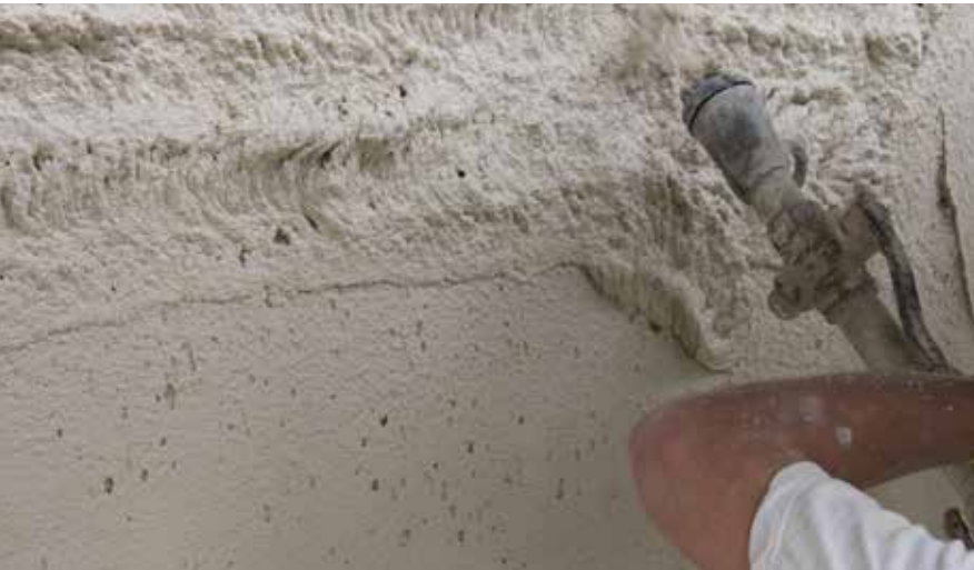
Figure 27: Machine application of insulating plaster. Wet-on-wet, thick-layer application © Fixit AG
