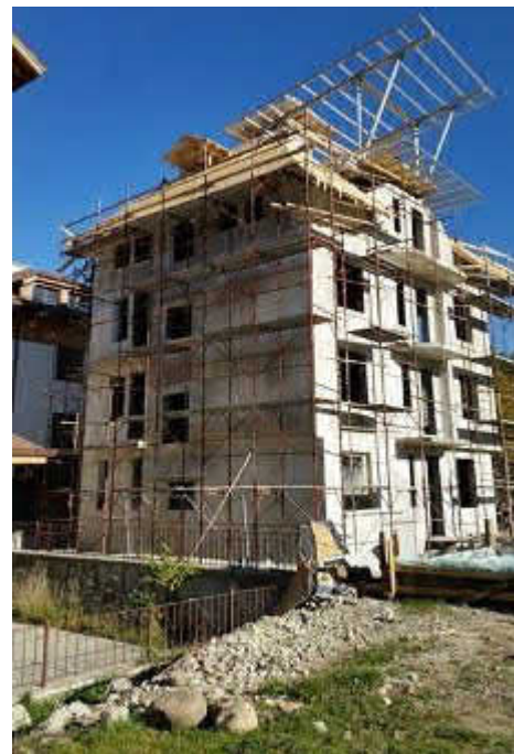
Figure 25 Building during construction works
