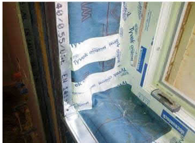
Figure 27 New airtightness seal by window
