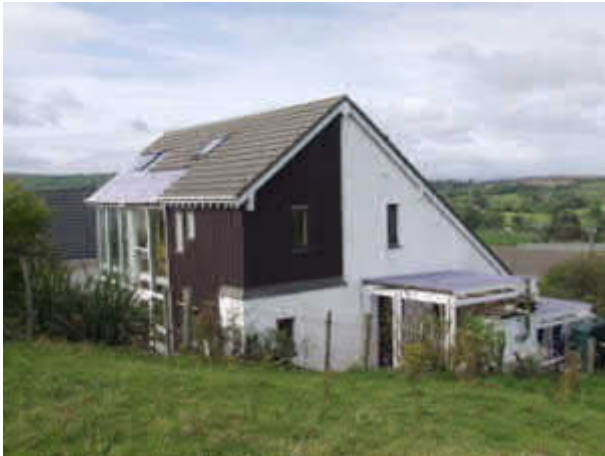
Figure 22 Building before retrofit measures
