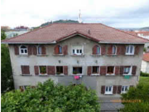
Figure 17 Building before retrofit measures
