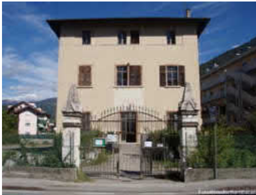
Figure 28 Building before retrofit works
