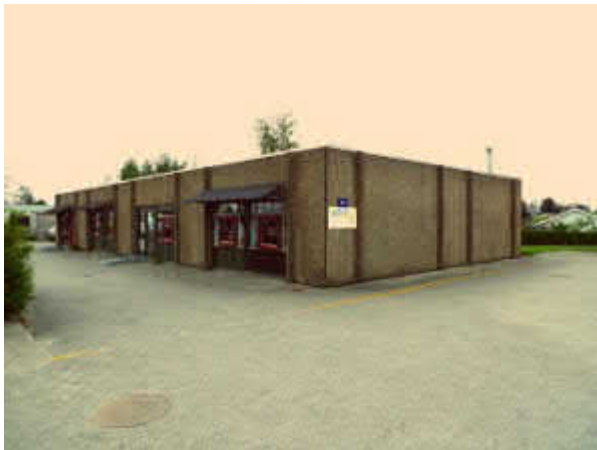
Figure 9 Building before retrofit measures
