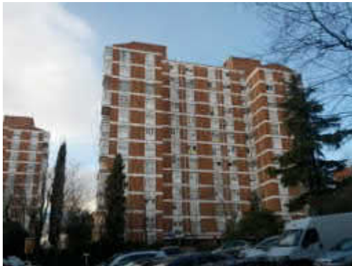
Figure 26 Building before retrofit measures
