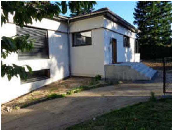
Figure 20 Building before retrofit measures
