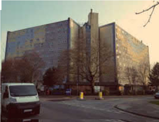
Figure 12 Wilmcote House before works
