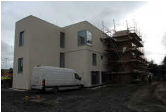
Figure 5 Northwest view showing site progress
