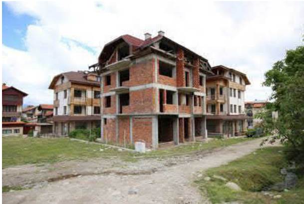
Figure 24 Building before construction works
