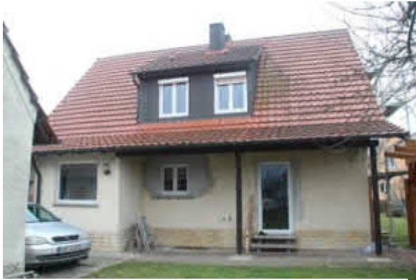
Figure 18 Building before measures
