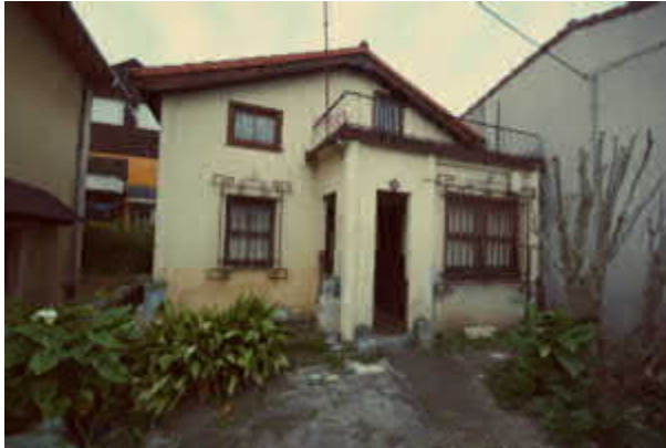
Figure 16 Building before construction work
