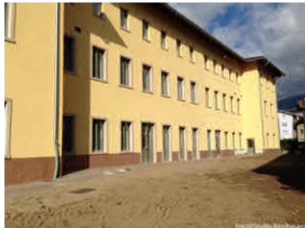
Figure 29 Existing building and extension
