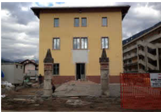
Figure 30 Building during retrofit works
