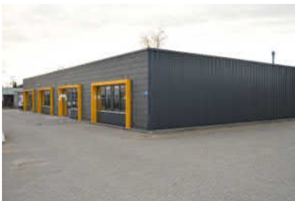
Figure 10 Building after façade insulation and window replacement
