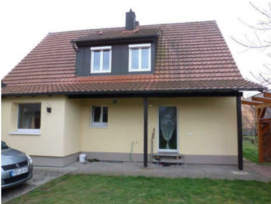
Figure 19 Building after measures
