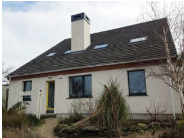
Figure 23 Building after retrofit step 1
