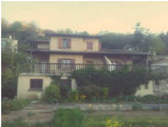
Figure 14 Building before construction work
