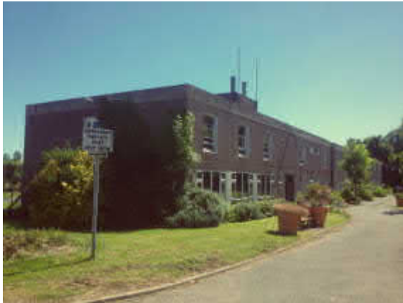
Figure 4: Northwest view of building before construction works
