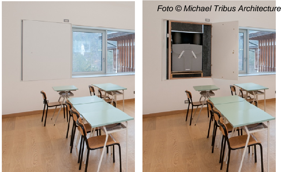
Figure 2: Ventilation device for a classroom integrated in an element of a curtain wall system [Source: Michael Tribus Architecture]
