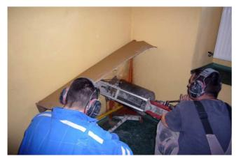
Figure 8: Most important part of installation – drilling of holes through the façade
